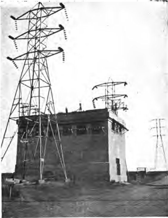
FIG. 203. Type of transmission lines used on the Big Bend-Oakland Line. Faccioli in the Trans. A.I.E.E.
